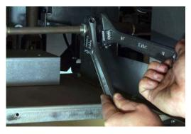
Holding backup while unscrewing flare nut on oil-return line.
